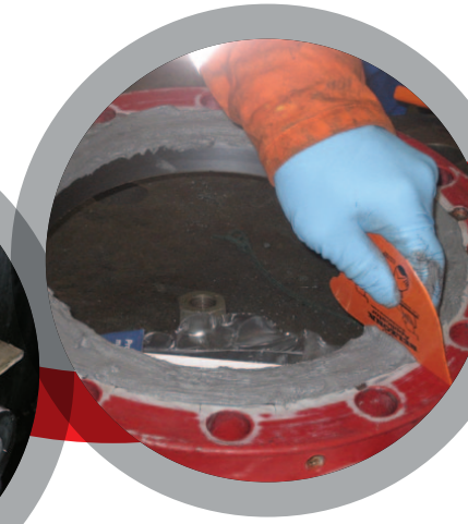
Flange Rebuilding
